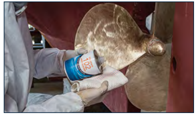
Clean surface with pure acetone.
